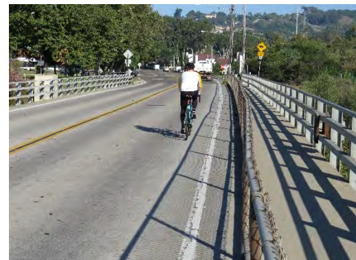
Existing bridge has lack of amenities for users
