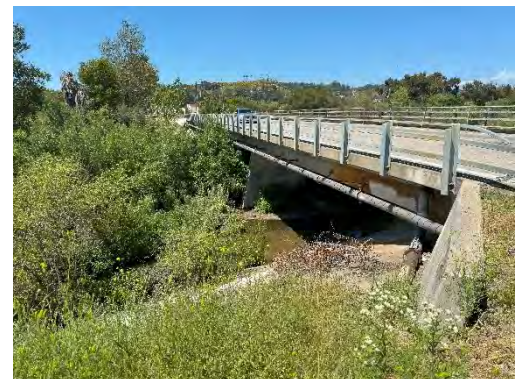
Westerly side of La Novia Avenue Bridge
