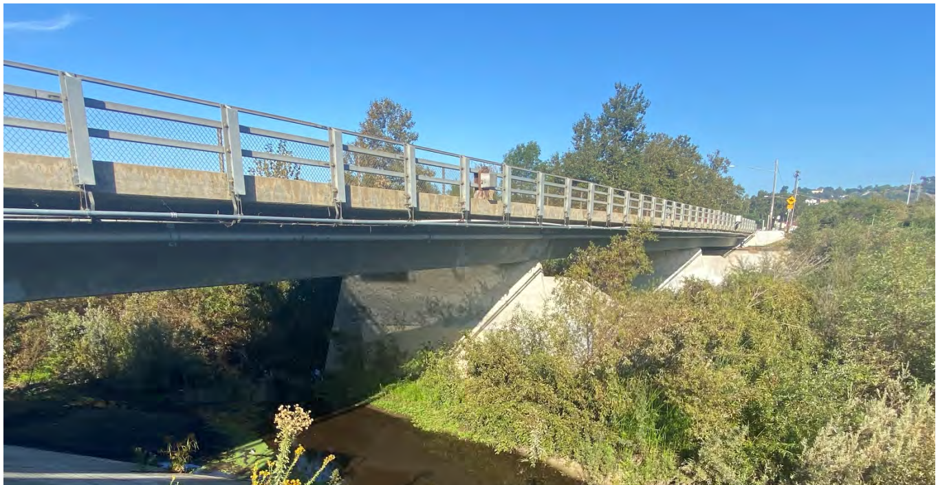
Existing La Novia Bridge over San Juan Creek
