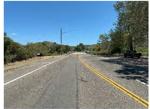
View of La Novia Avenue, Looking South
